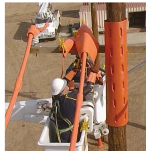
Strong memory improves grip when applied to the utility pole. The pole guard has high impact properties suitable for cold weather service.
