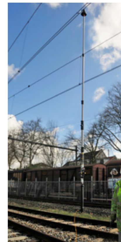
Test at a rail overhead line
