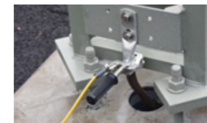
Earthing to grounding cable or fixed ballpoint with universal clamp (TT 36UK)
