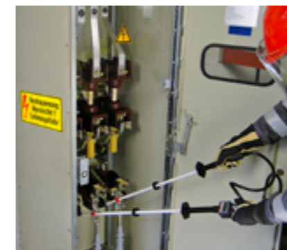
Test with HS 11 at 10 kV transformer
